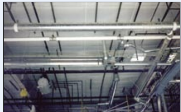
Example of things properly fastened to ceiling.
