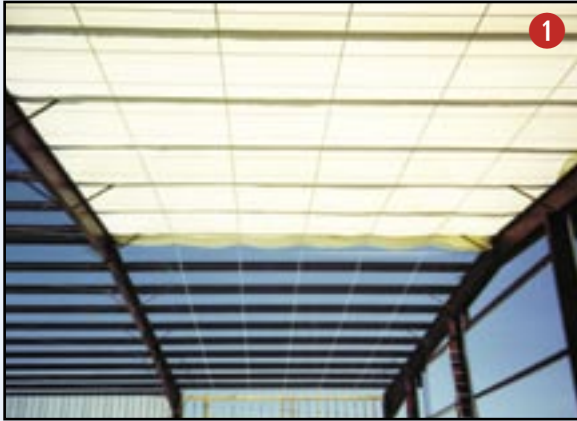
Large custom-sized ceiling fabric installs quickly on structural steel strap network.
