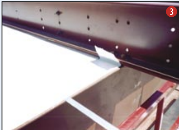
Ceiling fabric adhered to rafter for a sealed vapor retarder.
