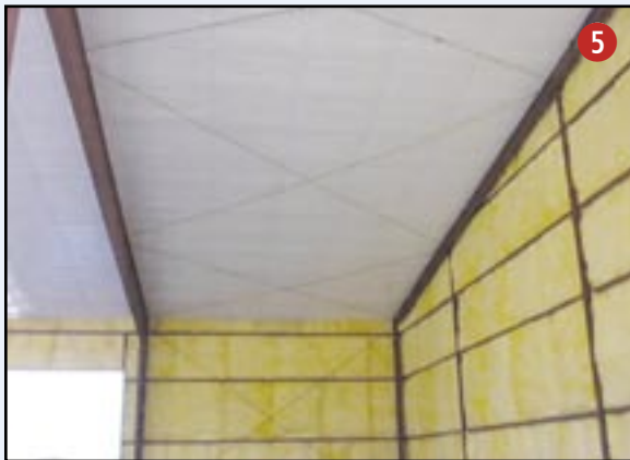
Full thickness insulation placed on wall and ceiling system.
